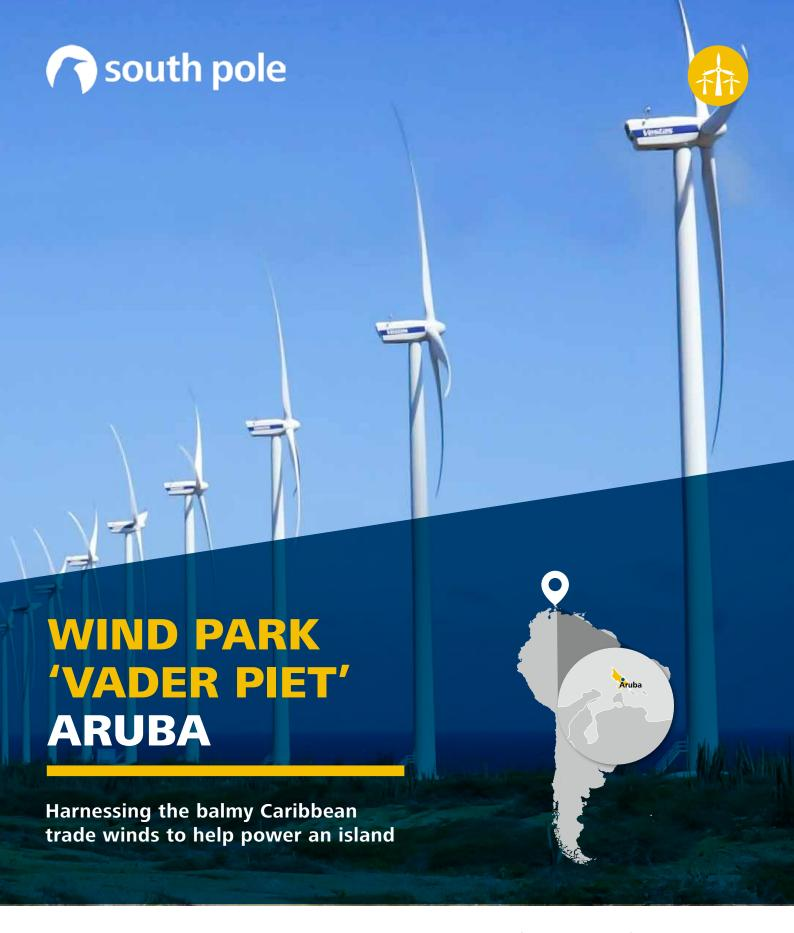
Located on Aruba's east coast in the Dutch Caribbean, this wind farm consists of 10 turbines and has a total installed capacity of 30 MW. Wind Park 'Vader Piet' supplies 126,000 MWh of electricity to the national grid each year, displacing fossil fuel-generated energy and supporting the island's transition towards renewable energy sources.
