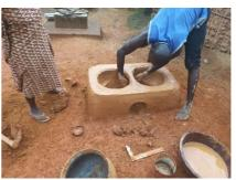
The in-situ multi pot stove has one combustion chamber and space for placing two pots for cooking. Following the Water Boiling Test (WBT) protocol, WBTs have been conducted by an independent consultant and a thermal efficiency of 21.7% was established in the case only one pot is used at the time, and 40.6% in case two pots are used for cooking at the same time.
